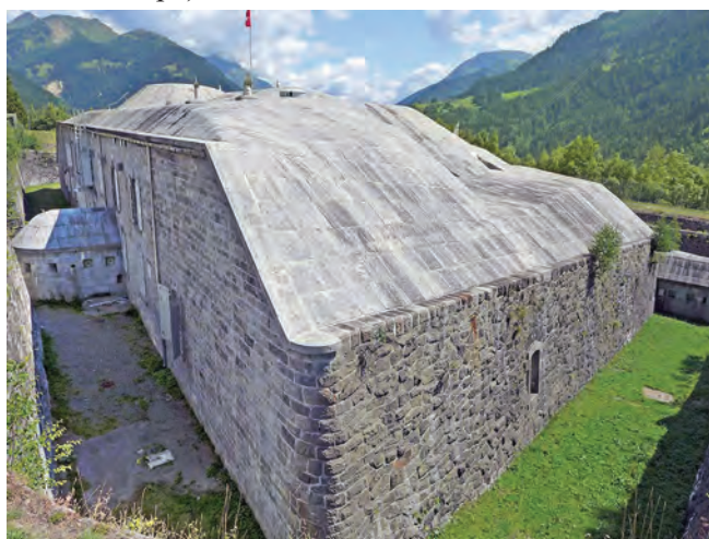
Fort Airolo: A classic late-19th century granite fort, built just as such structures were becoming vulnerable to rifled artillery firing explosive shells
